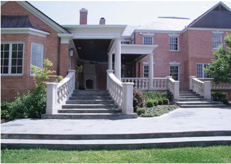
Left: The rear elevation AFTER renovation with new porch and basement level between bedroom wing to the left and addition to the right, re-whitewashed brick, and new terrace, pool, and outdoor dining pavilion (shown left) contrasts with the rear elevation BEFORE renovation (shown above) showing poorly spaced column configurations, proportionally heavy cast stone balustrade, stripped brick, and overall poor composition. Right: A new stair hall (right) connects the new garage level entry up to the renovated kitchen and new family room, and the bedrooms above.
